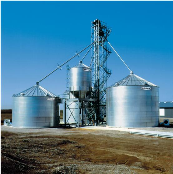
Tall structure in the middle is called a grain leg, angled components are fill augers
