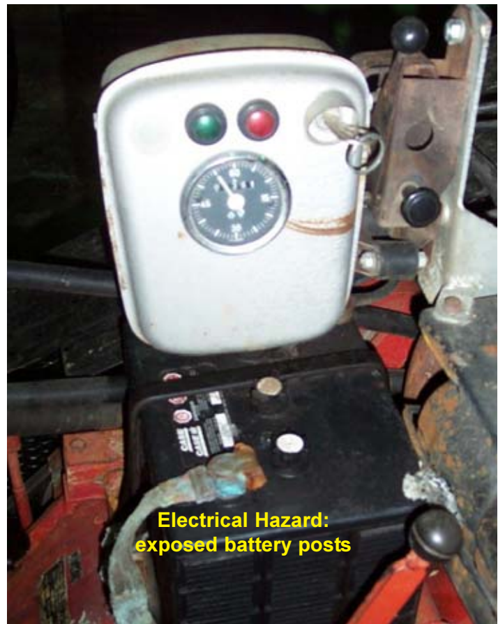
Figure 19. This electrical hazard could easily be eliminated by battery post covers or a battery box.
